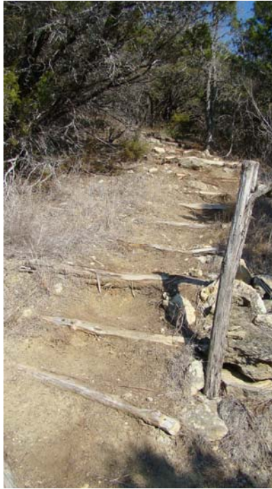
Figure 5: Erosion bars created from cedar to stabilize the hillside.
