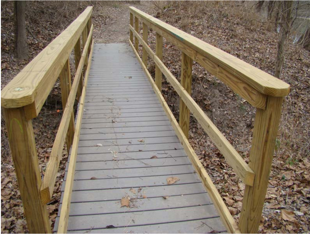
Figure 55: Recycled and Treated Lumber Boardwalk. Colorado River Refuge Bastrop, Texas
