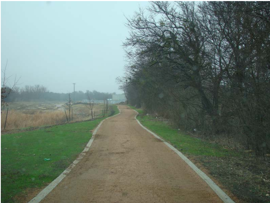
Figure 72: Granite Gravel with Ribbon Curb Trail. Round Rock, Texas
