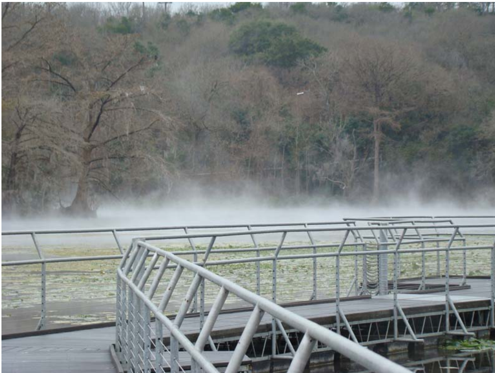
Figure 60: Floating Recycled Lumber Boardwalk. Texas Rivers Center. San Marcos, Texas
