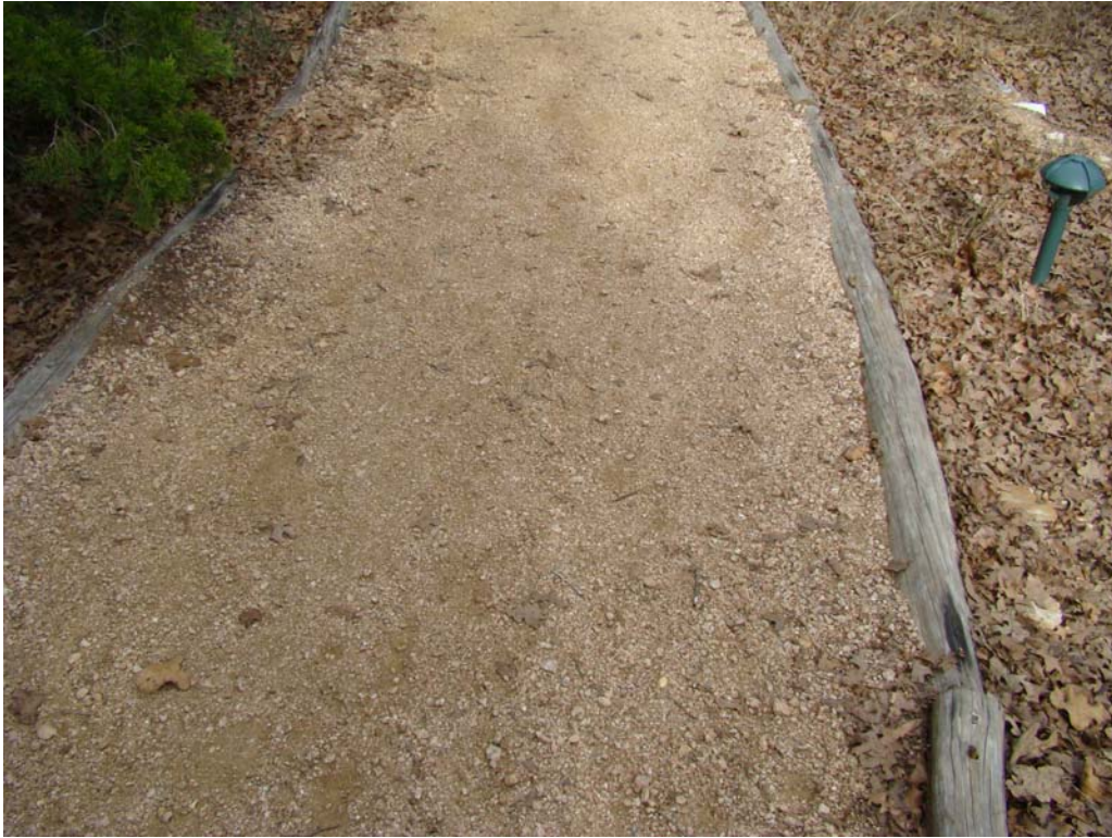
Figure 51: Granite gravel path with natural cedar border. McKinney Roughs Natural Area
