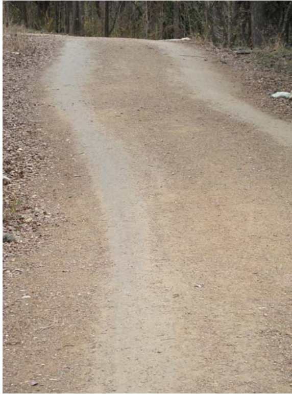
Figure 49: Granite gravel with stabilizing polymer. Pease Park Austin, Texas
