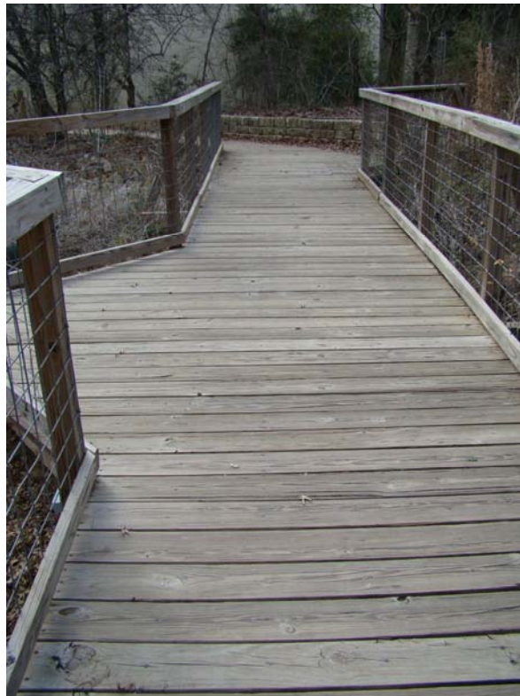
Figure 44: Boardwalk with rails made from treated lumber. Austin Nature Center.
