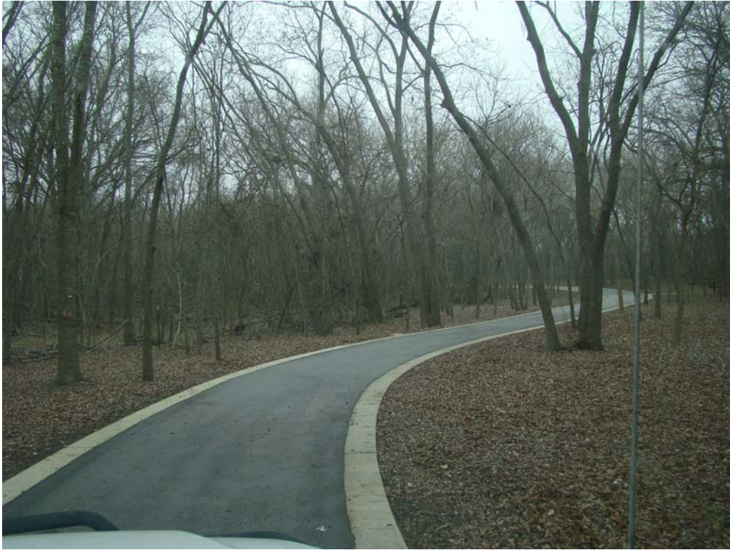
Figure 71: Asphalt Trail with Ribbon Curb. Round Rock, Texas
