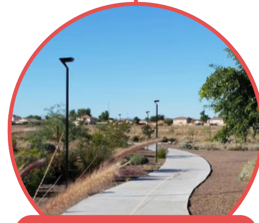
SOLAR POLE PATH LIGHTS
