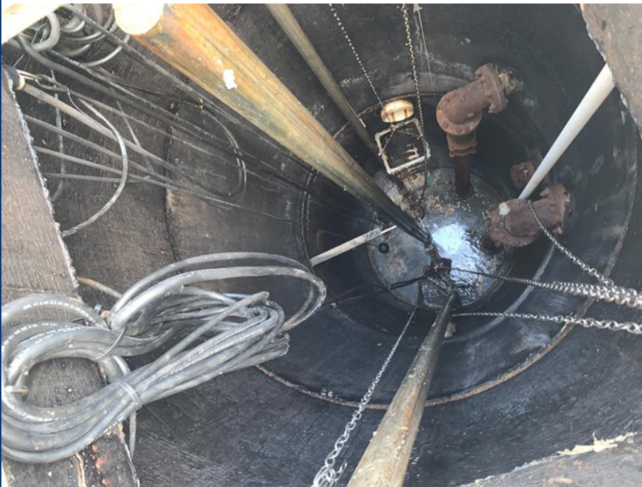
Inside of wet well (rails, float switches, pump pull chains, pipe and fittings, and debris baskets)
