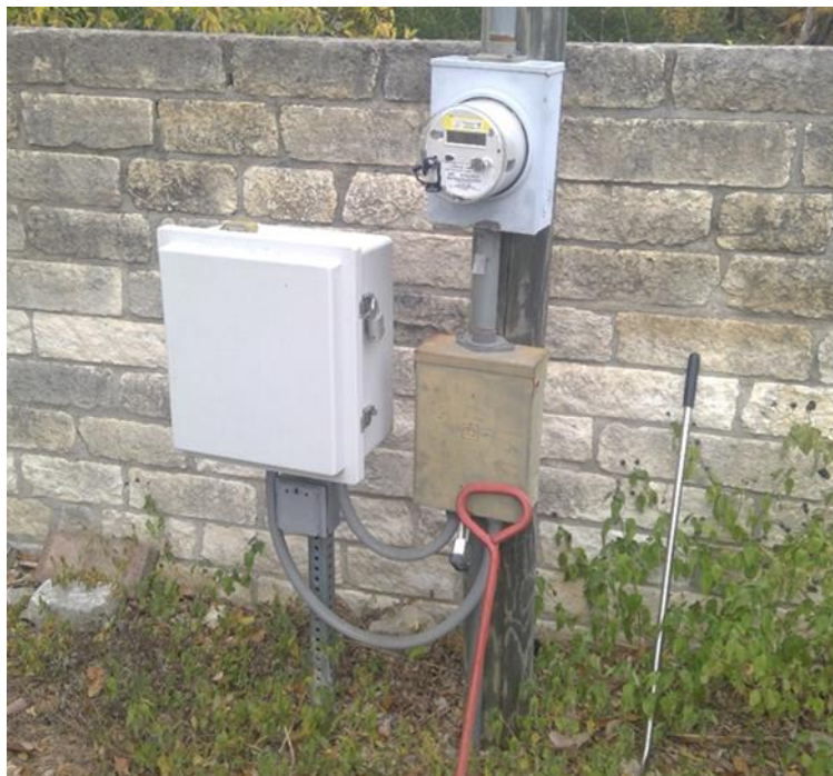
Service drop, meter, main power breaker, and generator connection
